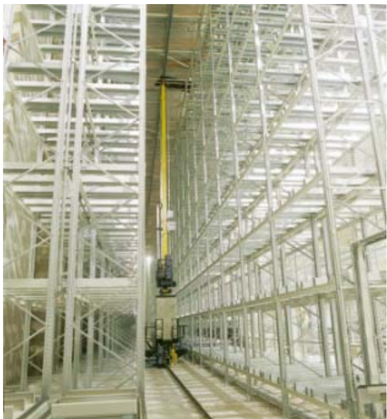
The logistic model of the new Kärsämäki factory includes an automatic high storage facility. Logistic flows are managed in real time from raw material purchases to targeted deliveries.
