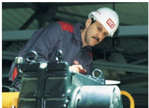
KCI Konecranes maintenance network also serves as an efficient distribution channel for other Group products. Professional maintenance services is the main driver for the Group's organic growth. In the picture Christian Banzet, service technician at Konecranes France.
