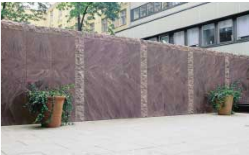
A natural stone wall built for Helsinki's Islamic congregation.
