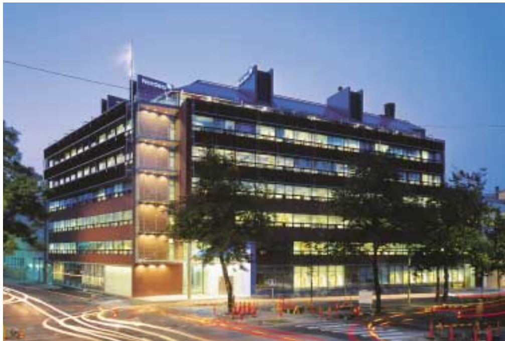
Lemminkäinen Construction Ltd's contract for Nordea's office building in the Vallila district of Helsinki was chosen as Environmental Project of the Year.
