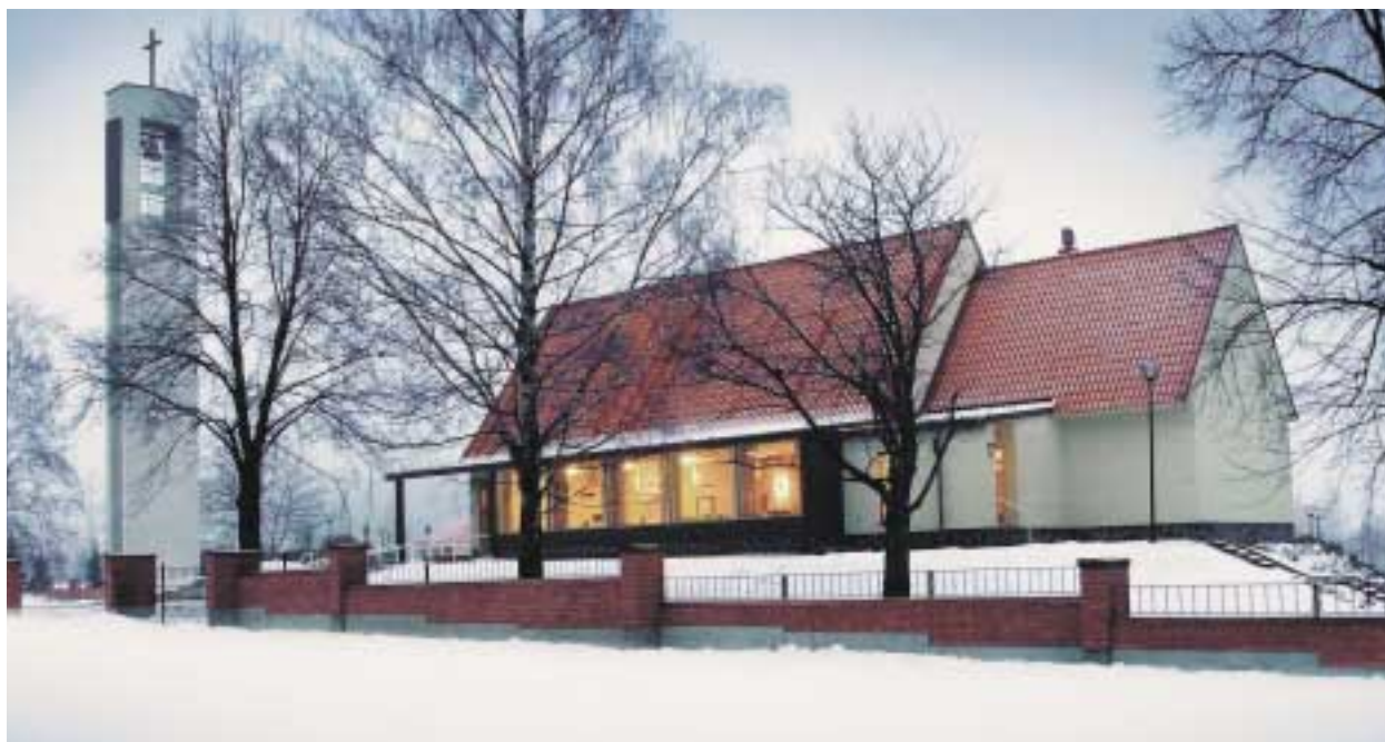
Laune church's clay tile roof, which was built by Lemminkäinen in 2001, was chosen as Roof of the Year.
