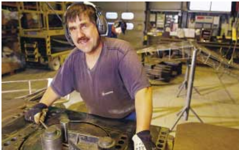
Paavo Kruut makes pre-cast concrete stair units at the Tuusula factory.
