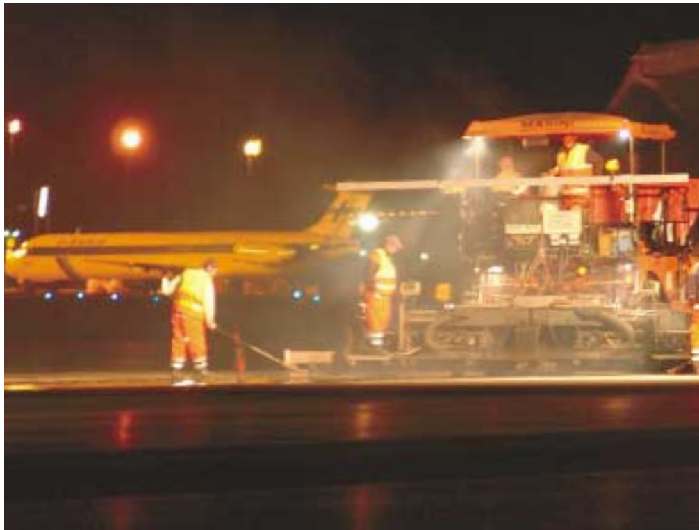
The runway at Oulu Airport was repaired in September 2001.
