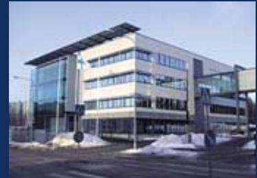
NCC has built no less than ten stages of the Tampere Technology Centre Hermia.
