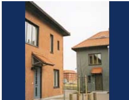
In the Kartanonkoski of Vantaa, an idyllic, Swedish-influenced housing village is under construction. The terraced houses of Eemeli and the Ritarla apartment buildings have already been completed.
