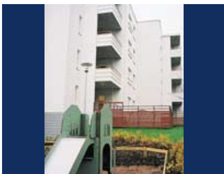
Kastehelmi in Espoo is a pastel apartment building in a spacious location on a hillside site.
