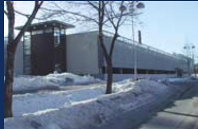
A car park was built for Tampere University of Technology. NCC improved the designs so much that the final result could accommodate 450 cars instead of the earlier 390.
