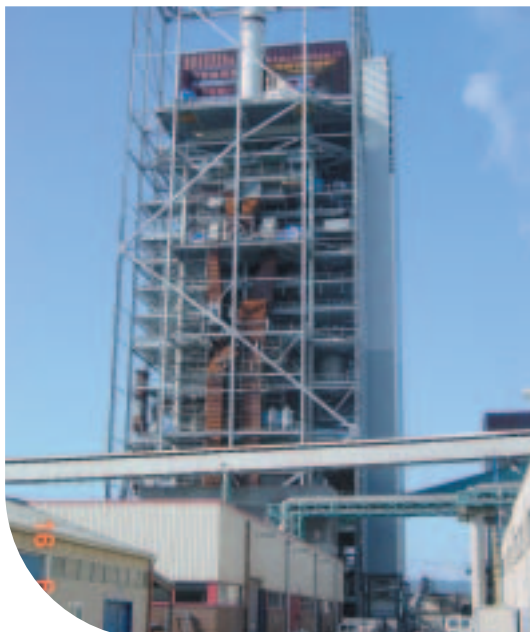
Recovery boiler plant, 2,000 tds/24 h, for Burgo Ardennes' ECP pulp mill in Virton in Belgium, supplied by Kvaerner Pulping Oy.
