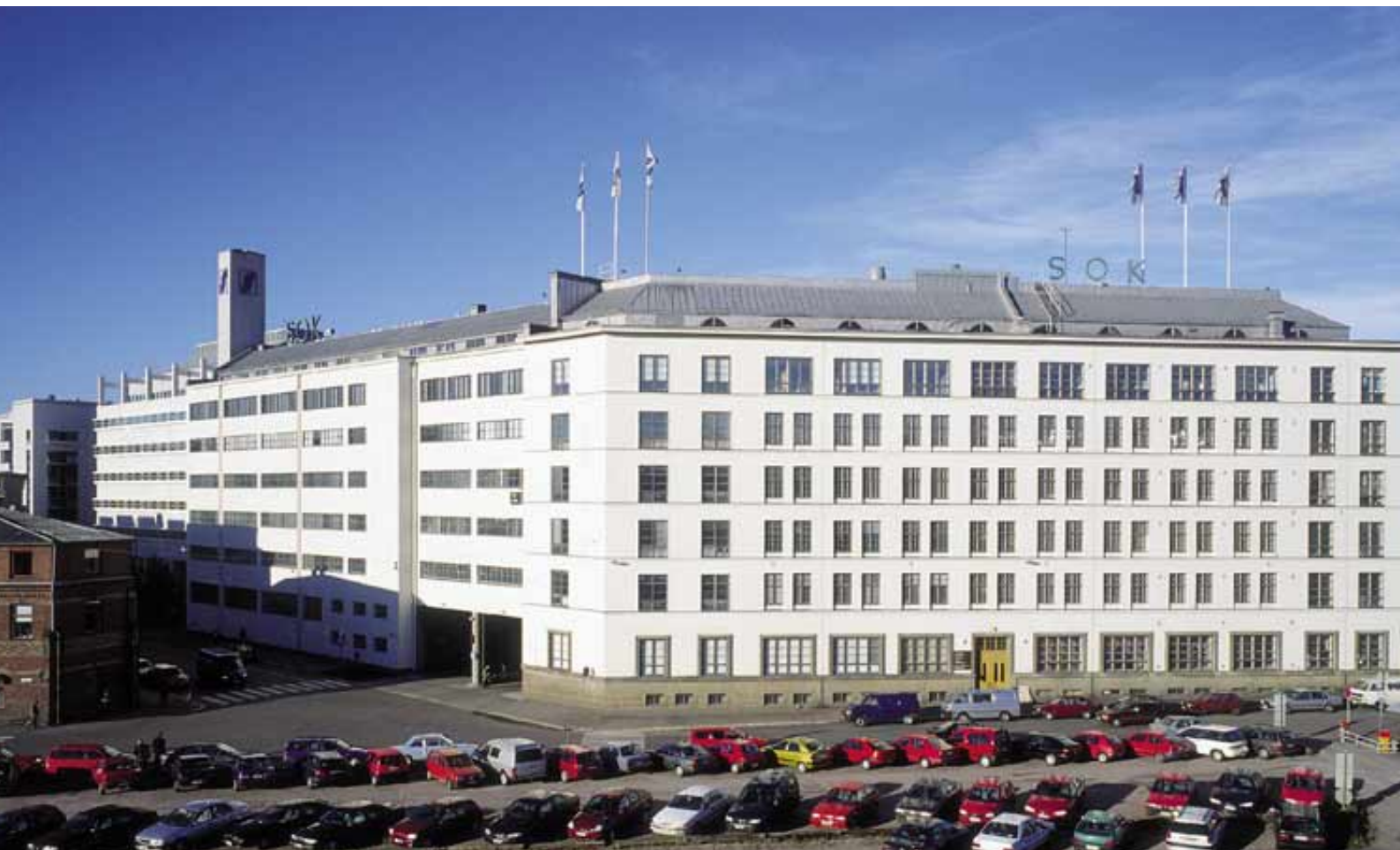
Vallila office block, Helsinki
