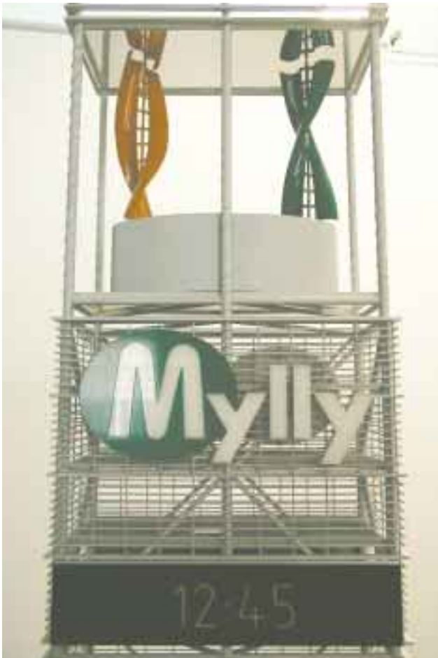
Spinning atop the 50 metre high tower at the Mylly shopping centre are two turbines whose energy output goes to the restaurants that enliven the shopping centre.
