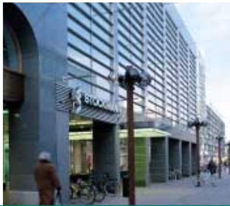
The Oulu department store spans the block and opens on to four streets. This is the stylish view on the Kauppurienkatu side.
