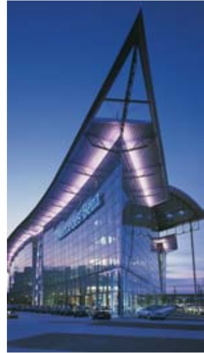
Velta Contec heating and cooling system was installed in the 'Mercedes World' building in Berlin, Germany.
