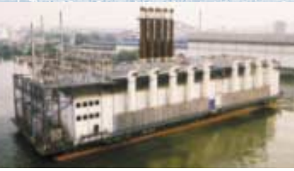
The world's largest floating power plant, Sultana del Este.
