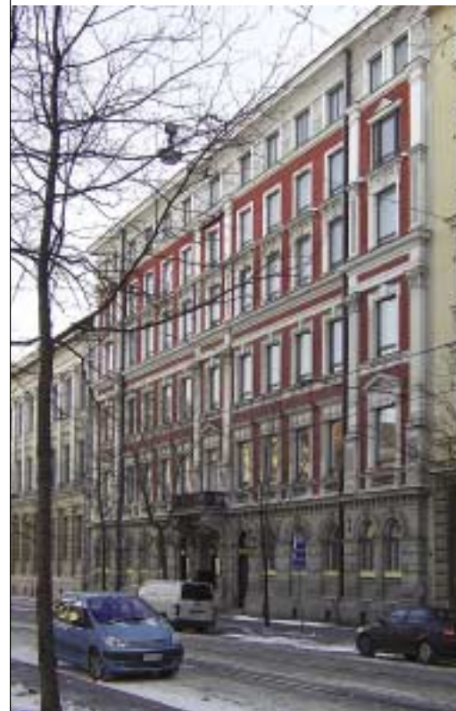
The renovation and extension works on the Mandatum Bank were completed in Helsinki.
