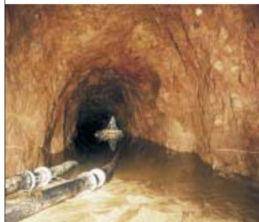
28 kilometres of the Päijänne tunnel were refurbished.
