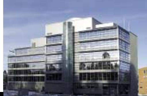
LPG Innovations Oy's office building in Espoo.
