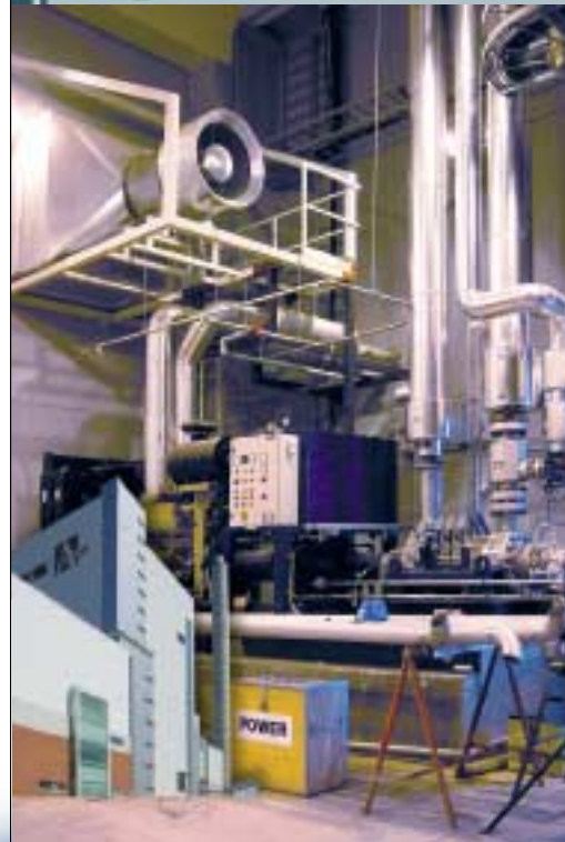
Photos above: Alholmens Kraft in Pietarsaari is the world's largest bioenergy plant. Its electrical output is 240 MW, or about one-fifth of the output of a nuclear power plant. YIT supplied high-pressure and primary low-pressure piping for Alholmens Kraft.
