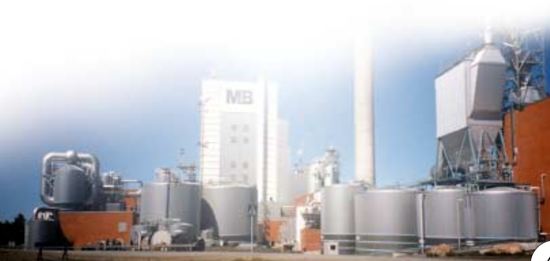
Photos above: Alholmens Kraft in Pietarsaari is the world's largest bioenergy plant. Its electrical output is 240 MW, or about one-fifth of the output of a nuclear power plant. YIT supplied high-pressure and primary low-pressure piping for Alholmens Kraft.
