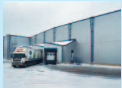
KWH Freeze, Huurre Finland Oy ▶
