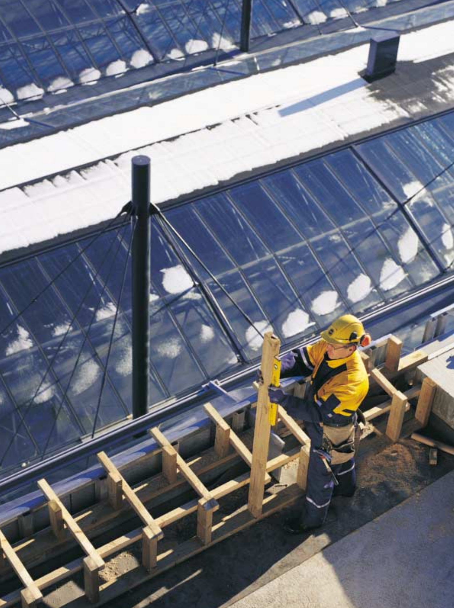
Carpenter Pauli Virtaniemi on the Eliel Hotel site in Helsinki.
