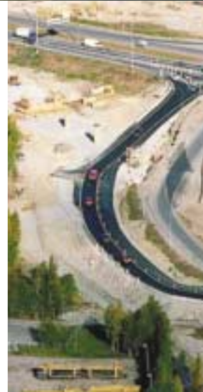
A major road building contract began on Ring Road III.
