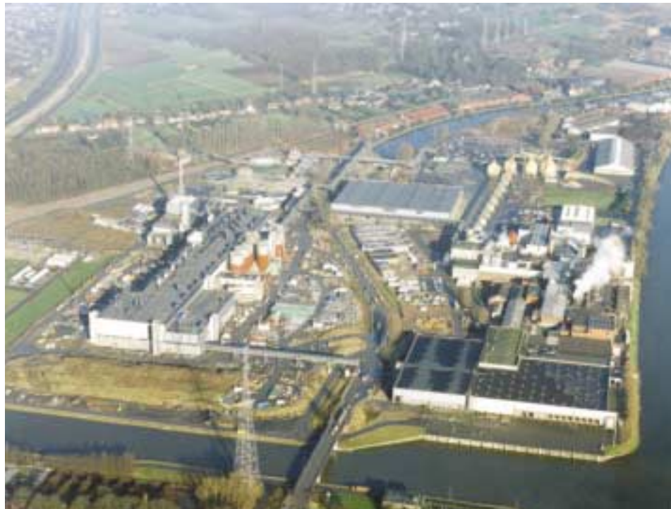
The biggest construction site abroad was Stora Enso's new paper mill in Gent, Belgium.
