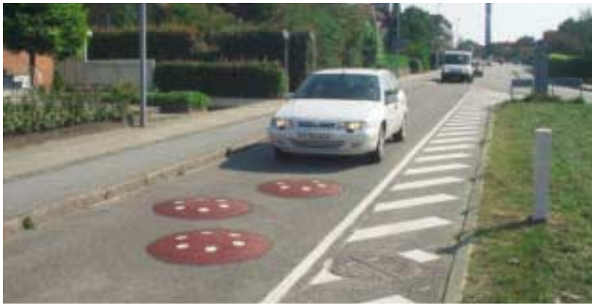
Lemminkäinen AS in Denmark has developed "Mushrooms" to control urban traffic, while allowing the unfettered movement of commercial vehicles. This patented product is undergoing trials in other countries as well.
