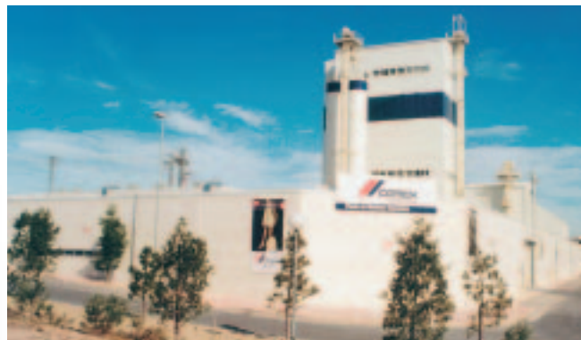
The project delivered to Spain in 2002 is Raute Precision's biggest single plaster and mortar plant sale so far.
