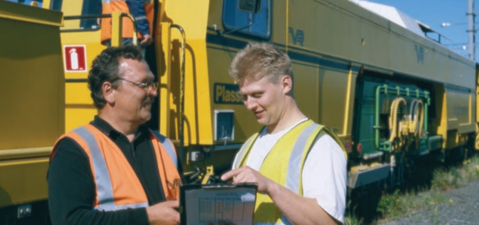
Track machinery is highly automated because the work demands speed and accuracy. The crew of this tamping machine includes foreman Jukka Makkonen and machine operator Jukka Latva.
