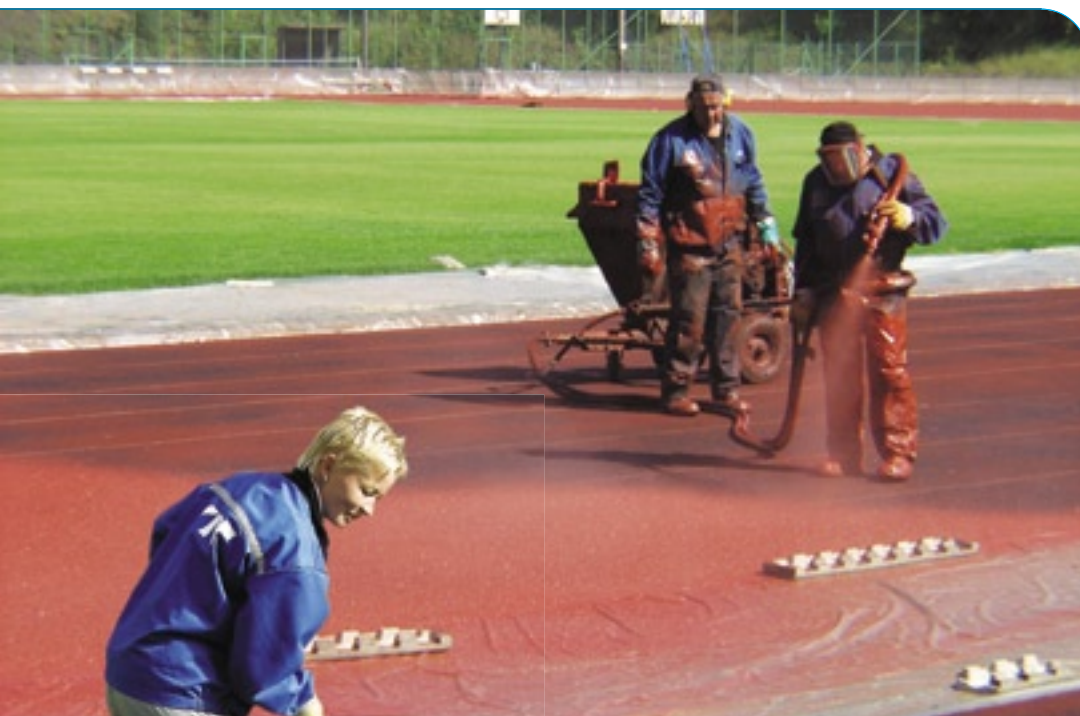
Tartan surfacing works on the running track of the Hiekkaharju track and field arena.
