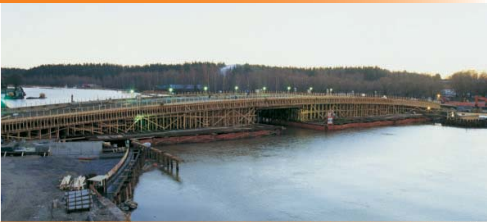
Aleksanterinkatu bridge in Porvoo before major concrete castings were made.
