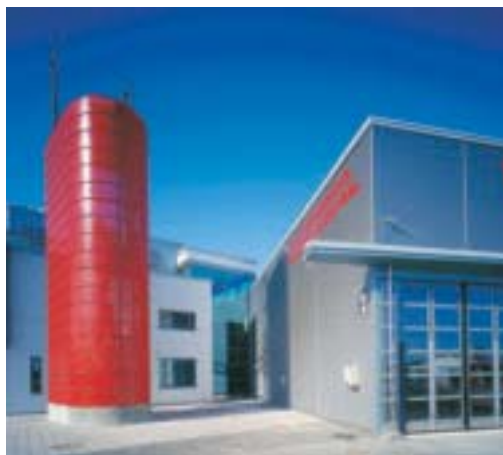
Tekmanni installed the technical building services for the rescue centre at Helsinki-Vantaa Airport.
