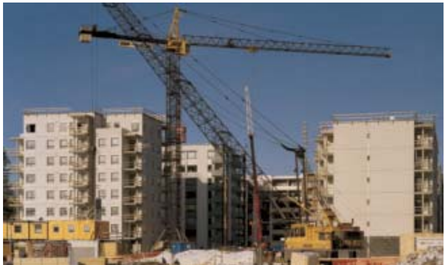
Palmberg's housing developments near completion in Espoo.
