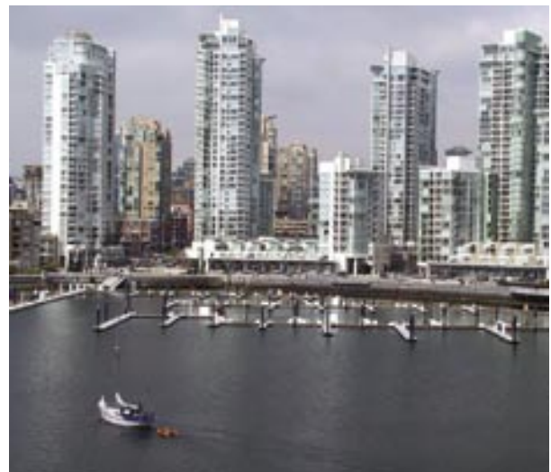
The Concord Pacific Vista residential and office towers in Vancouver, Canada, are plumbed with Wirbo AquaPex systems.
