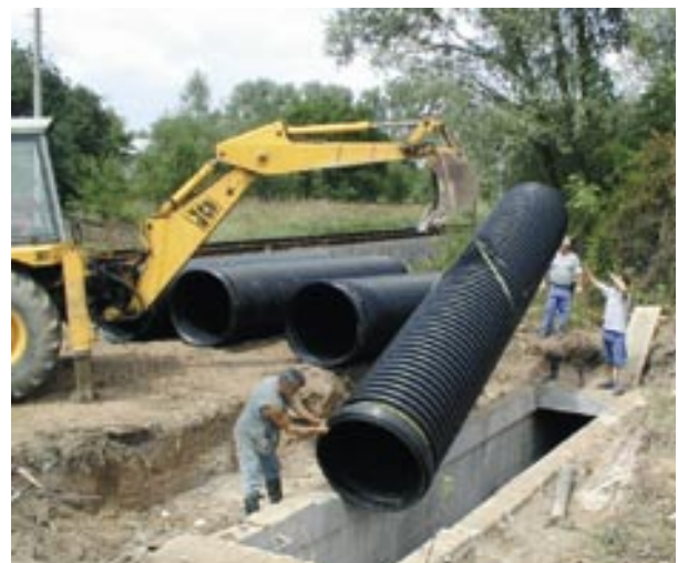
The wastewater network in the Czech Republic is renovated by the Uponor sewer pipe system.
