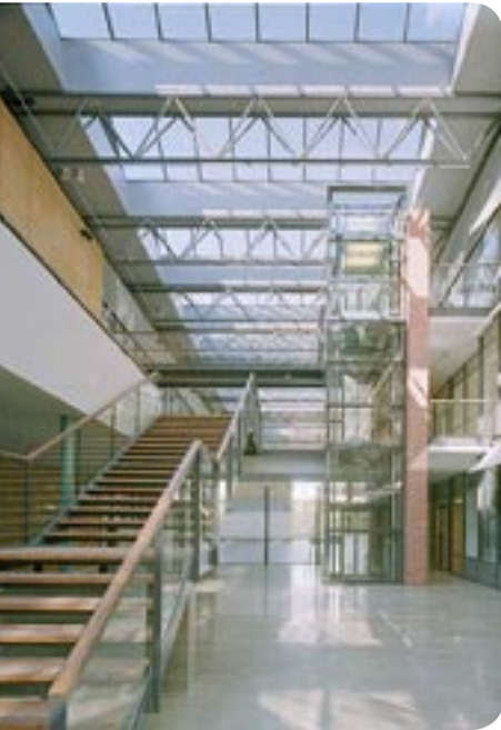
The Helsinki University of Technology's TUAS building was one of the pilot sites of Tekes' Terve Talo (Healthy House) development project.
