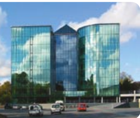
The Valdo deep-freeze storage facility and office complex in Riga
