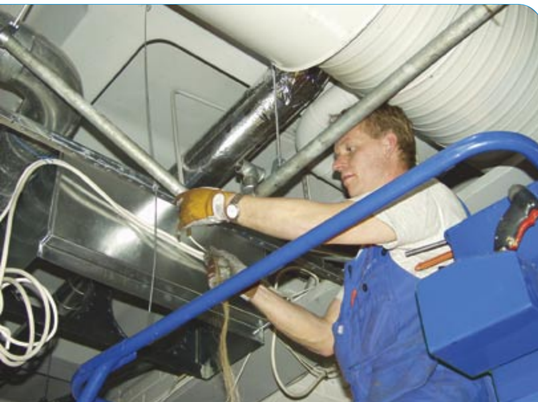
Electrical installer Reima Sintonen at the Hansa quarter site in Turku
