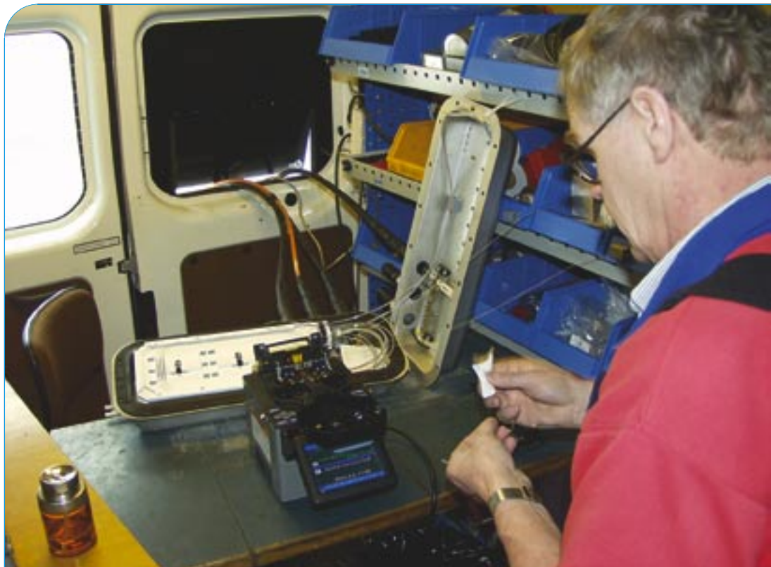
Telecom installer Jukka Ruokonen performing optical cable welding in the field
