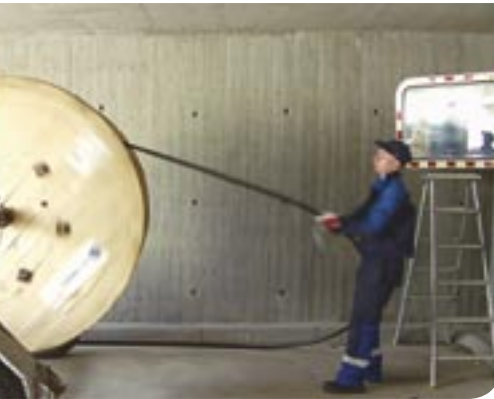
Telecom installer Timo Nikkanen installing copper cable
