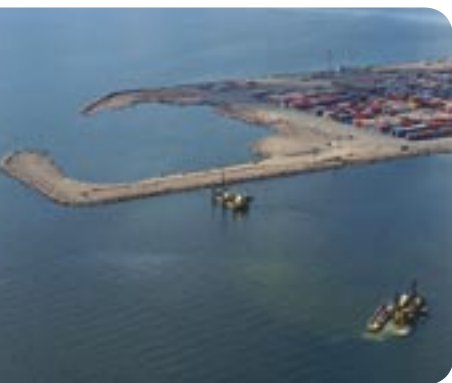
Extension of pier C at the Mus-salo harbour in Kotka
