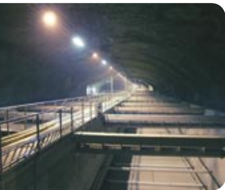
Interior finishing works at the Viikki wastewater treatment plant in Helsinki
