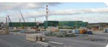
YIT built a sawmill in Pestovo for ZAO Pestovo Novo.
