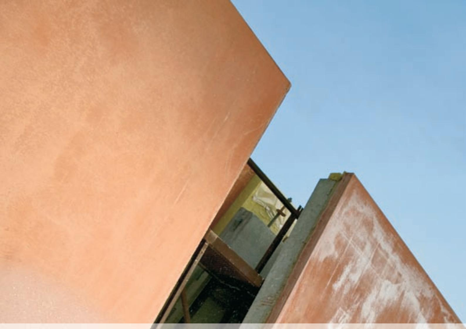
*Concrete elements do not have to be grey or dull. New technologies allow the use of different colours and textures.*
