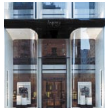
Asprey store in Trump Tower, New York, is a magnificent example of the use of safety glass.
