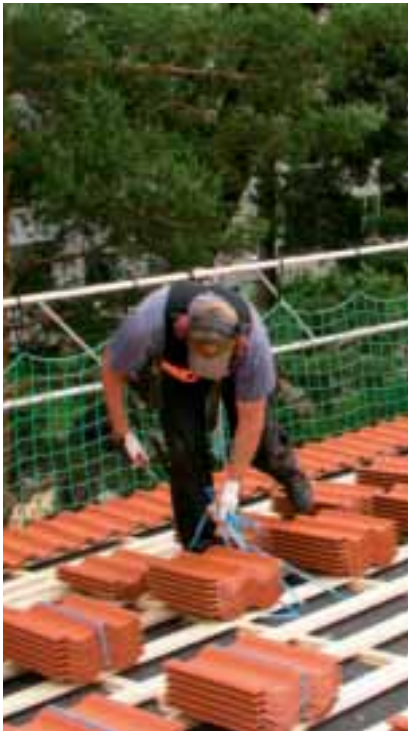
Properly installed safety rails protect both employees and members of the public.
