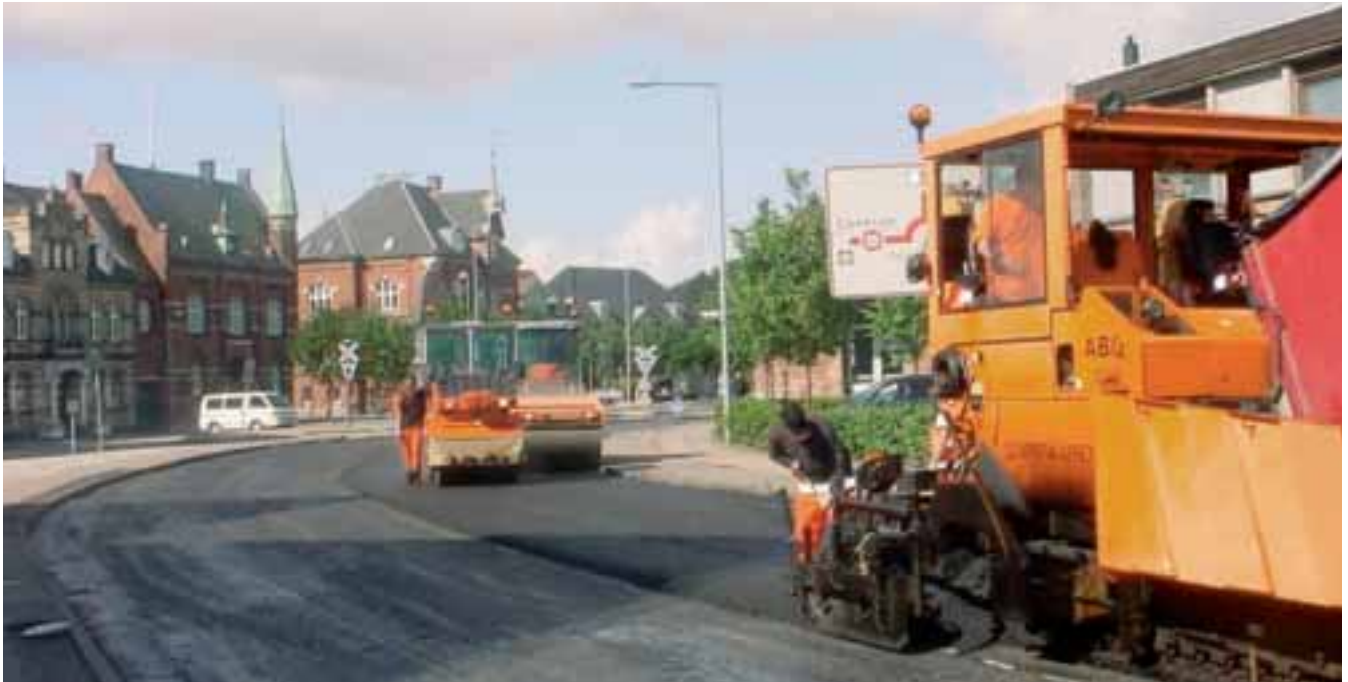
Street paving work in the harbour area of Vejle in Denmark.
