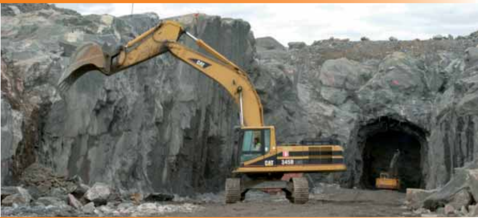
Lemcon Ltd is building Olkiluoto nuclear power plant's feed and return water channels together with their tunnels.
