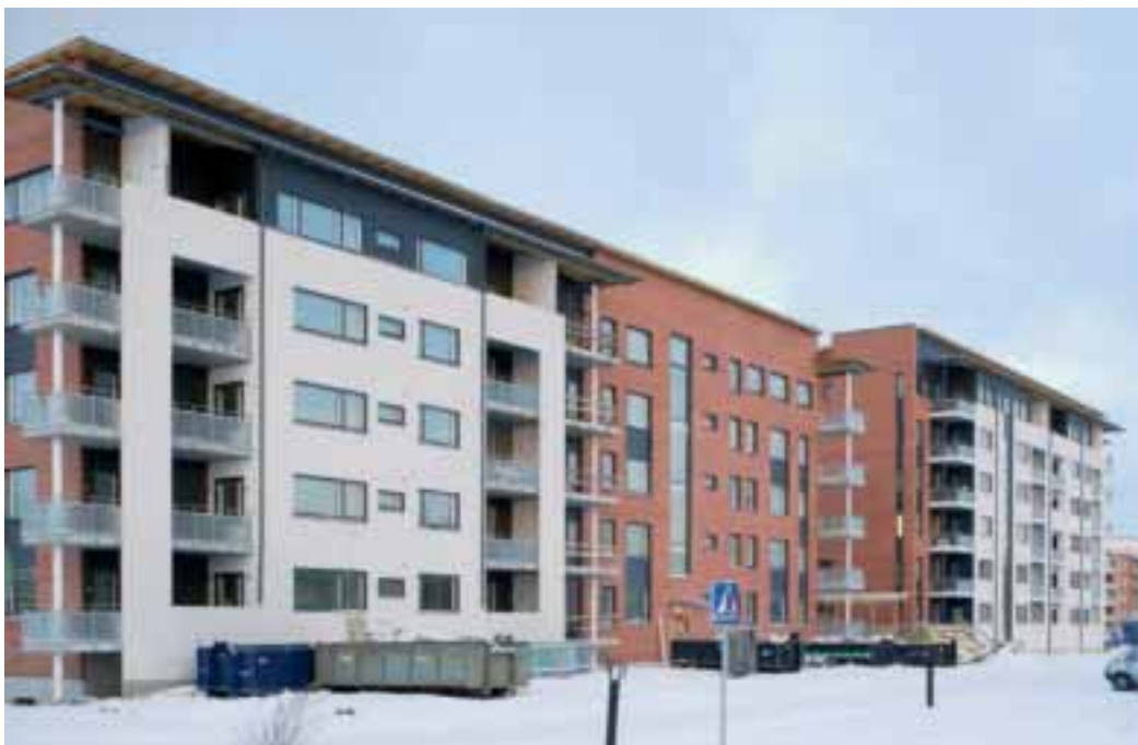
Palmberg-Rakenus Oy built new apartment buildings for YH and VVO Group in the Aine district of Oulu.
