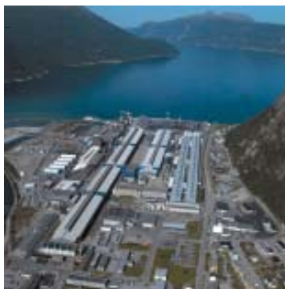
The picture shows the new Sunnalsöra aluminium mill of Norsk Hydro, one of Onninen's customers in Norway.
