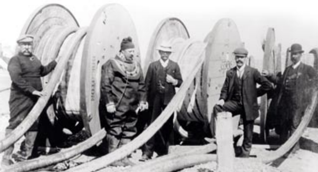
A team of Siemens employees laying a submarine cable in the 1860s
