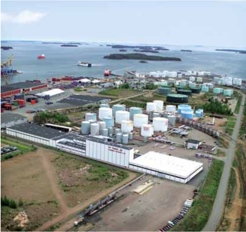
The lubricants plant, Hamina.
