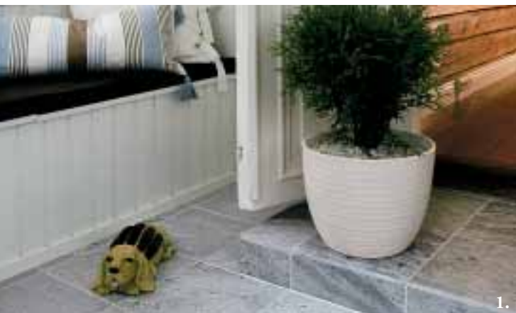
1. Soapstone is an excellent flooring material because it does not clatter, it retains the heat and it is not slippery even when wet.
