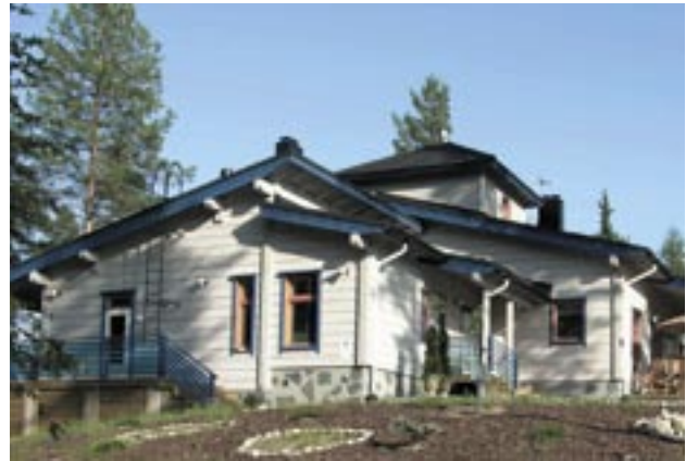
A one-family log house on display in the Finnish Housing Fair was completed on the lake waterfront in the summer of 2004. Concerned with the immediate surroundings and water system, the family opted for Uponor's biological-chemical wastewater treatment plant. The house uses geothermal heating, which distributes heating evenly thanks to radiant underfloor heating. Clean indoor air is guaranteed by a ventilation system, whose hygienic plastic ducts neither absorb dust nor let it circulate in indoor air. The system features a humidity sensor and heat recovery function, which protect the house and save energy. The house serves as a good example of Uponor's wide range of solutions considering that it supplied not only underfloor heating and ventilation systems but also tap water, sewerage and rainwater sewer systems.
