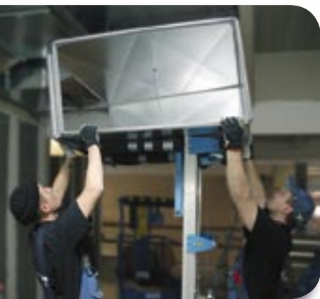
Ventilation installation works in the project to build business premises for the Finnish Meteorological Institute and the Finnish Institute of Marine Research in Helsinki.
