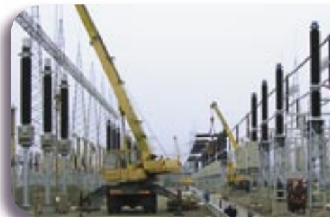
Eesti Energy is building a new switching substation in Narva.
