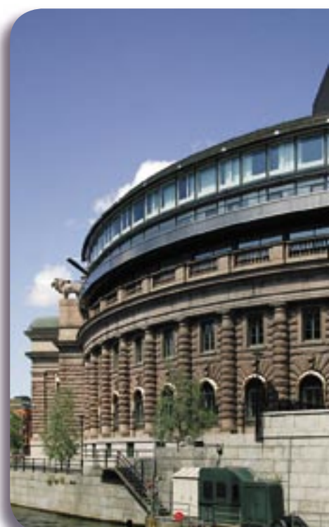
YIT is supplying a new security system for the Parliament of Sweden's buildings in Stockholm.
