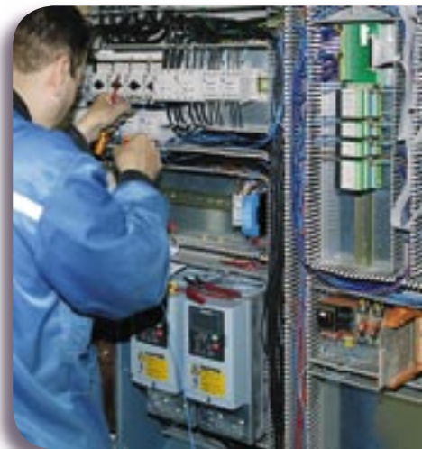
Automation installation at YIT's servicing point in Vantaa.
