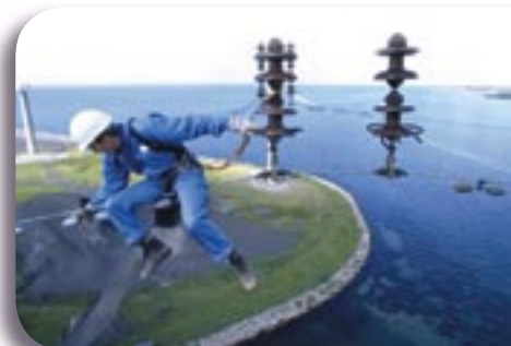
Power line servicing in Denmark.
