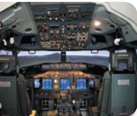
YIT is delivering electrotechnical installation works, ClimaCeil and piping works for SAS Flight Academy at the Gardemoen Airport in Oslo.
