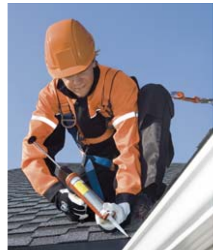
Roofer Janne Karjalainen at work on Kanava Golf's clubhouse in Vääksy.
