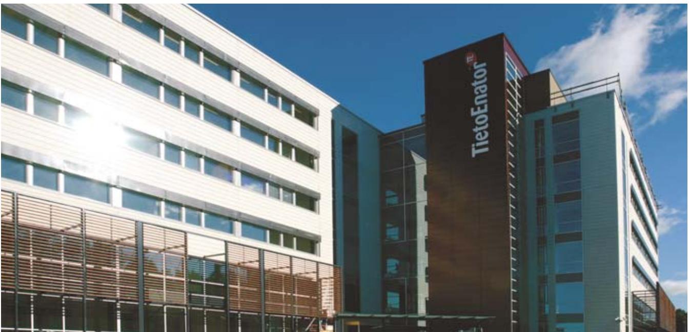
Almost 6 000 sprinklers were installed in TietoEnator's office building.
