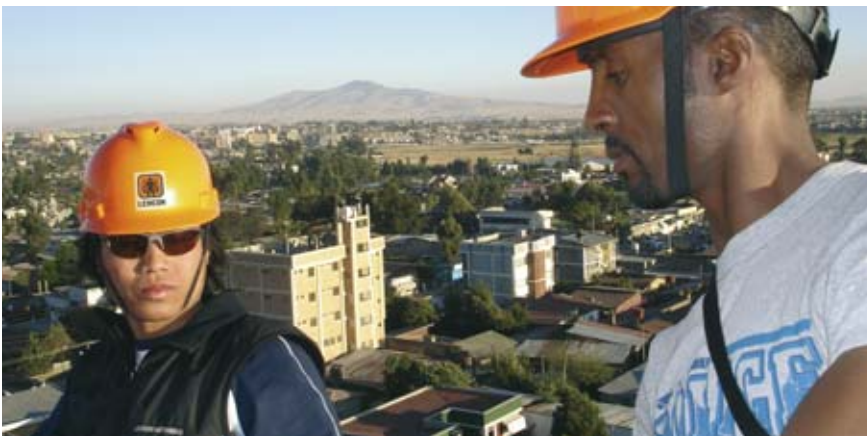
Engineer Giovanni Gorda and supervisor Yedenekachew Dessalegn on a telecom network installation site in Addis Ababa, Ethiopia.
