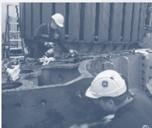
RENOVATION WORK IN KIERIKKI
