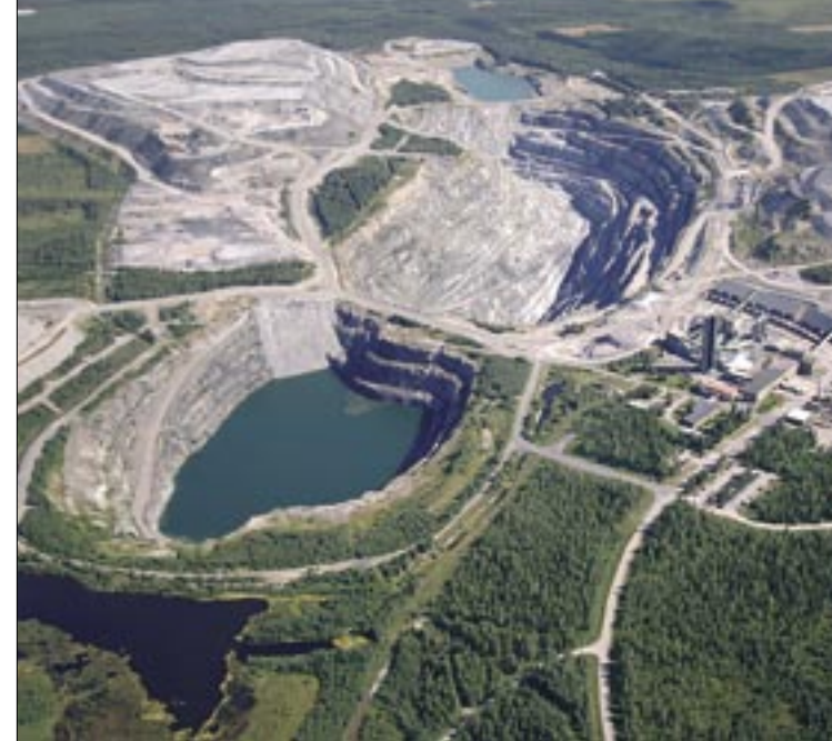
The excavation of tunnels for Outokumpu Chrome Oy got under way in Kemi at the only chrome mine in the EU countries.
