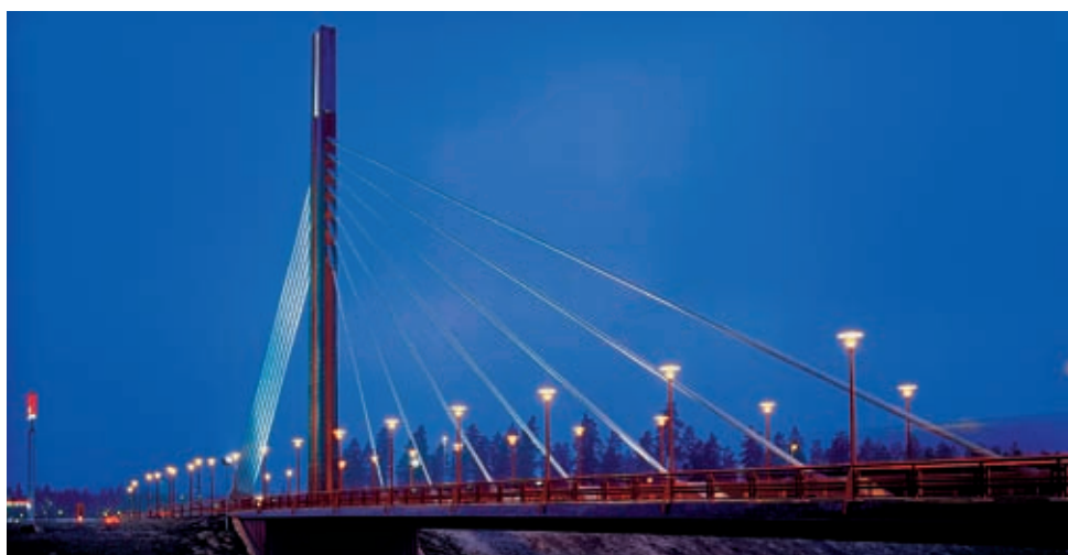
Forssan Betoni supplied the ready-mix concrete for the Lippo bridge on Highway 3.
