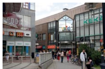
Trio Lahti Citycon's gross leasable area 43,900 sq.m. Built in 1987. Extended and/or renovated in 1992/2007/2008.
