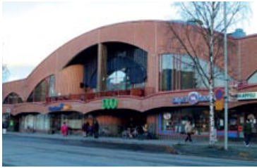
Duo Tampere Citycon's gross leasable area 13,000 sq.m. Built in 1979. Extended and/or renovated in 2007.
