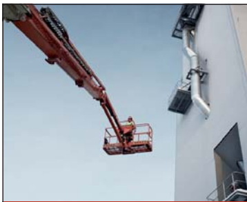
AERIALS AND FORKLIFTS
