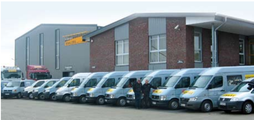
The new service centre of the German Ponsse distributor Wahlers Forsttechnik GmbH in Stemmen.
