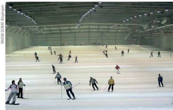
The most modern skiing hall in Europe, Snow Dome in Bispingen, Germany, can accommodate up to 4,600 skiers per hour in the slopes cooled by Uponor solutions.
